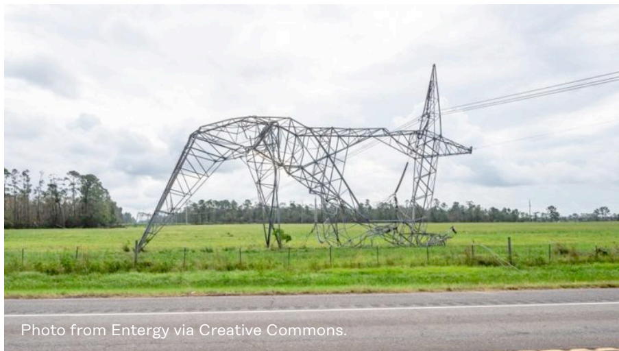
Figure 9. Damage from Hurricane Laura on overhead transmission
