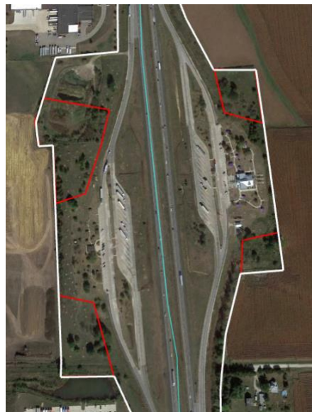
Figure 8. Example rest area showing potential area for solar PV installations outlined in red
