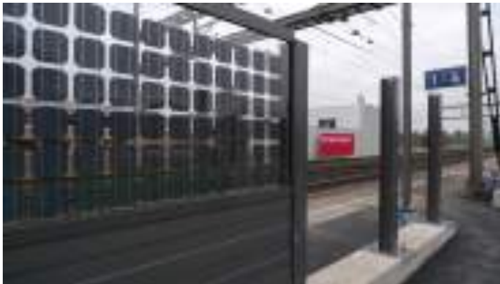
Source: TNC Energie
